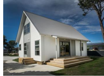
Fraser Street show home
